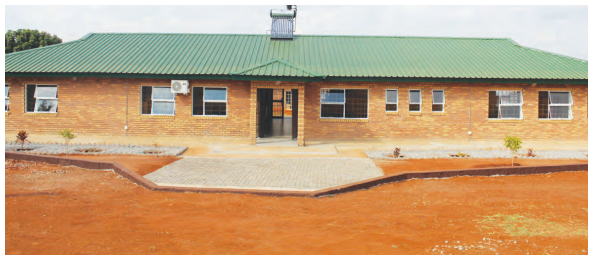
The new administration block that was handed over to Hlakanang Primary School by Twickenham Mine in July 2023.
