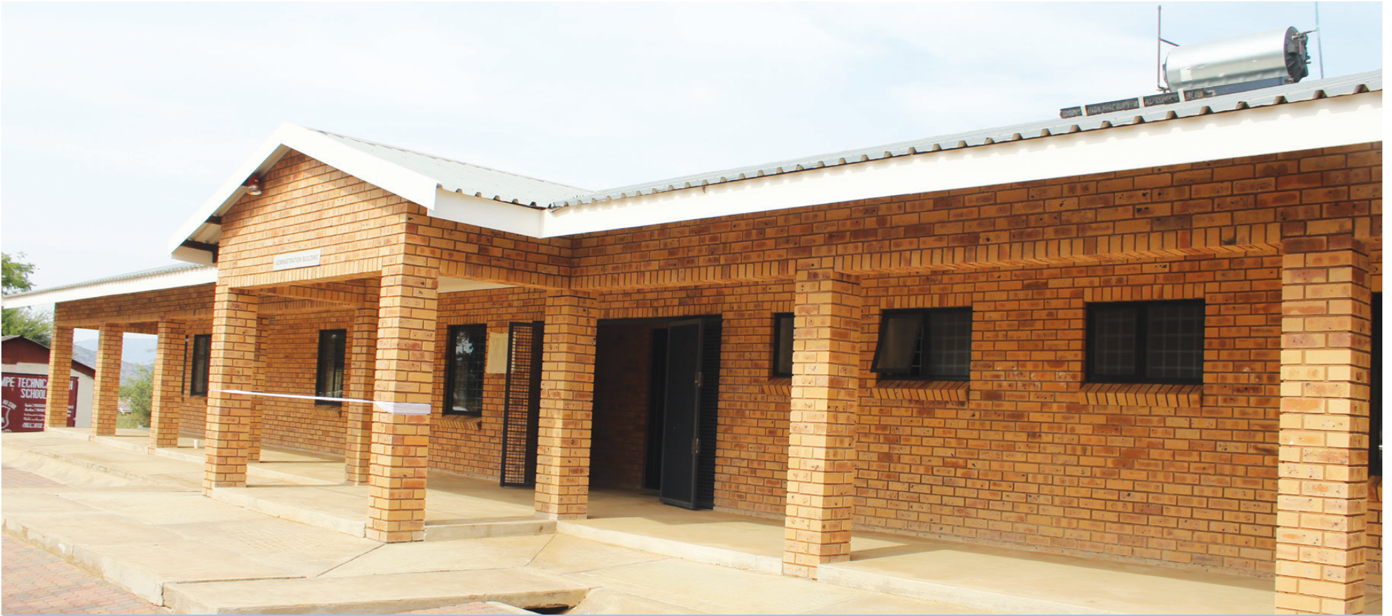
Identical administration blocks were donated to Makgopa Primary School and Ntoampe Technical High School.
